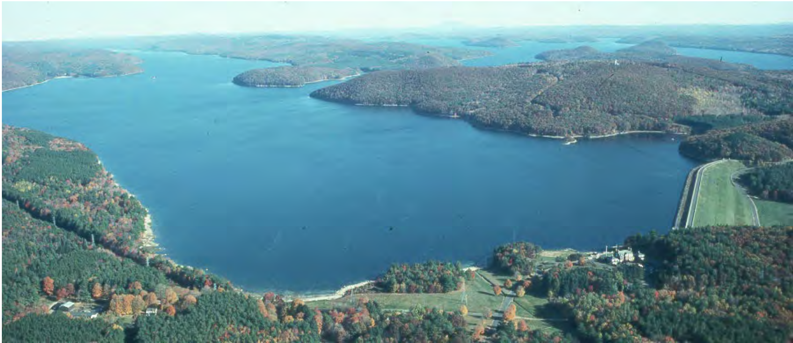
Quabbin Reservoir and Winsor Dam, Swift River, MA, 1946 (massmoments.org) 170 ft (52 m) high, 412 billion gallons of water storage (1.56 km 3 )
