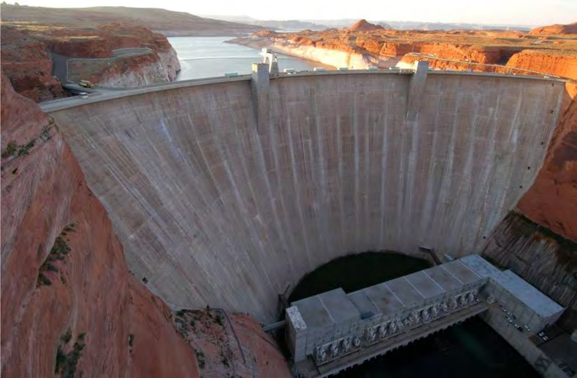
Glen Canyon Dam, Colorado River, AZ/UT 316 m tall, 32 km 3 of storage, 1300 MW power generation
