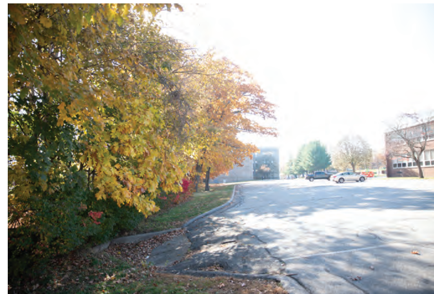
School parking lot with drainage problems.
