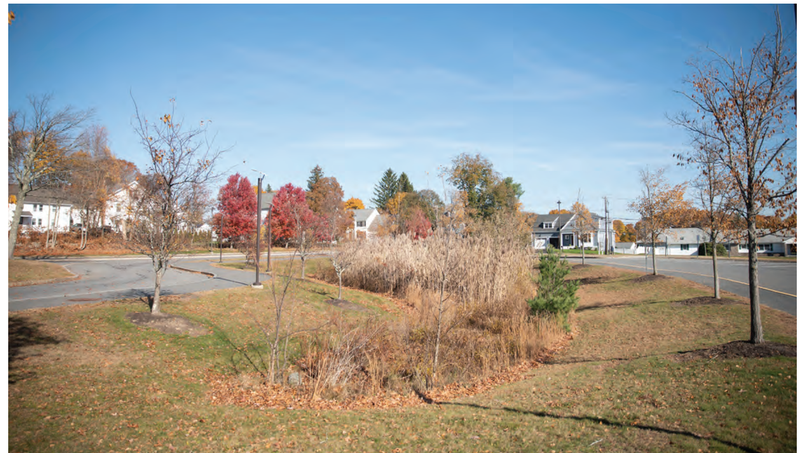
Current stormwater treatment system in front of Brookside Elementary School.
