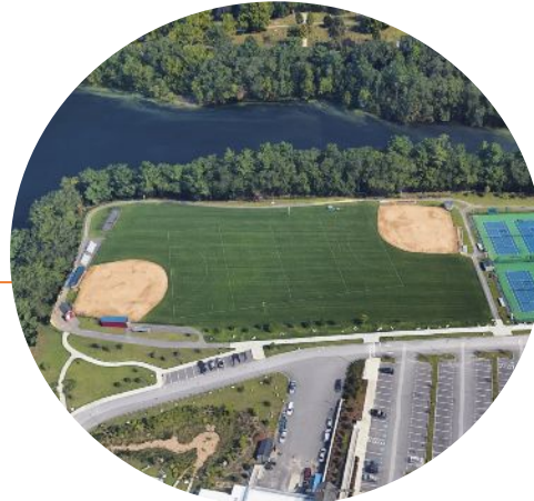
Subsurface storage underneath playing field
