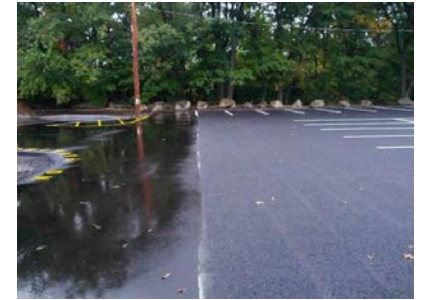
With Porous Pavement
