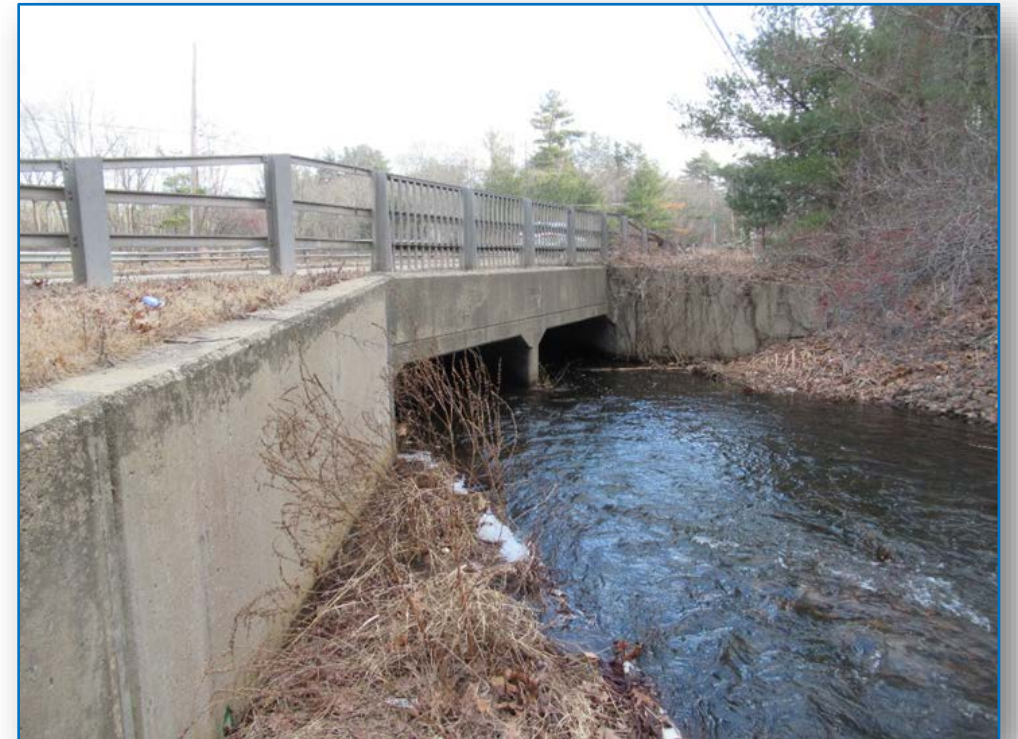
Upstream view of Rt 140 crossing (twin 8 x 4 ft box culverts)
