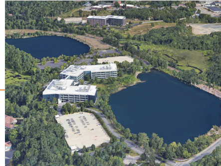
Retention Pond Retrofit
