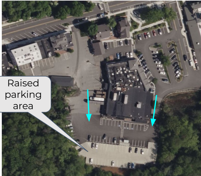
Frequent flooding occurred at the southern end of the parking lot, in 2019 Weston raised that section
