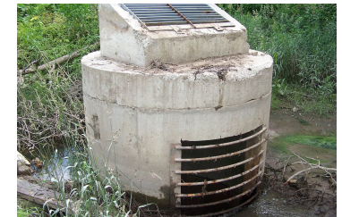
Outlet Control Structures
