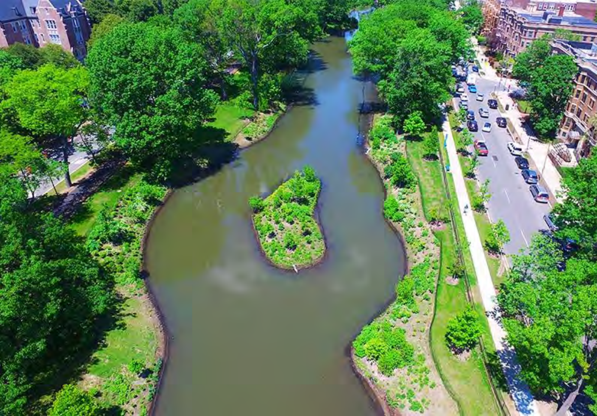
Aerial of Muddy River Restoration Area
